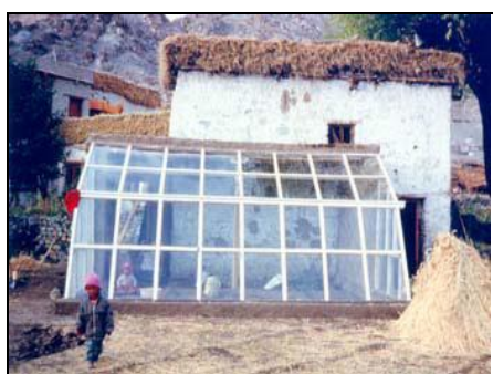
Figure 5: A passive solar house with thermal insulation reduces the cost of heating by 90% (GERES Afghanistan)
