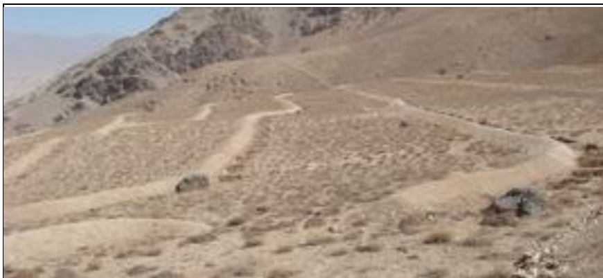
Figure 3: Contour trenches with continuous bunds (HELVETAS Swiss Intercooperation Afghanistan, 2015)
