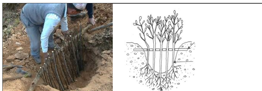
Figure 11: Construction of palisades (Shrestha et al., 2012)
