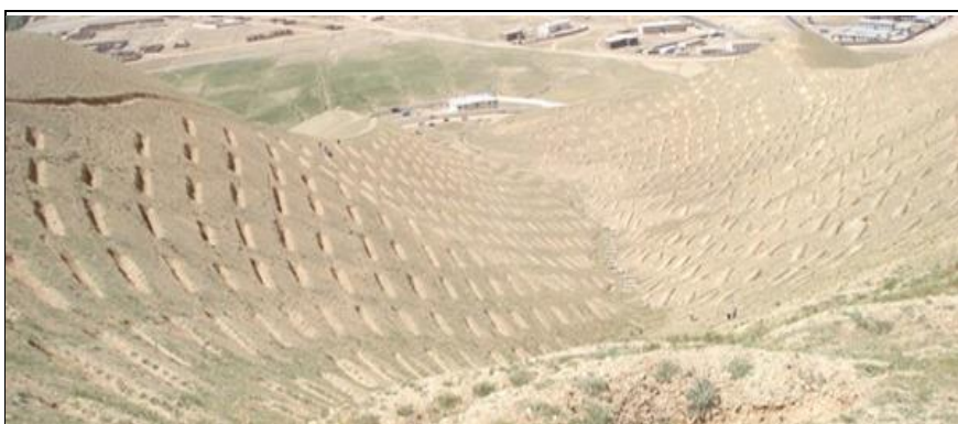
Figure 4: Contour trenches with a staggered design (HELVETAS Swiss Intercooperation Afghanistan, 2015) WOCAT sheet
